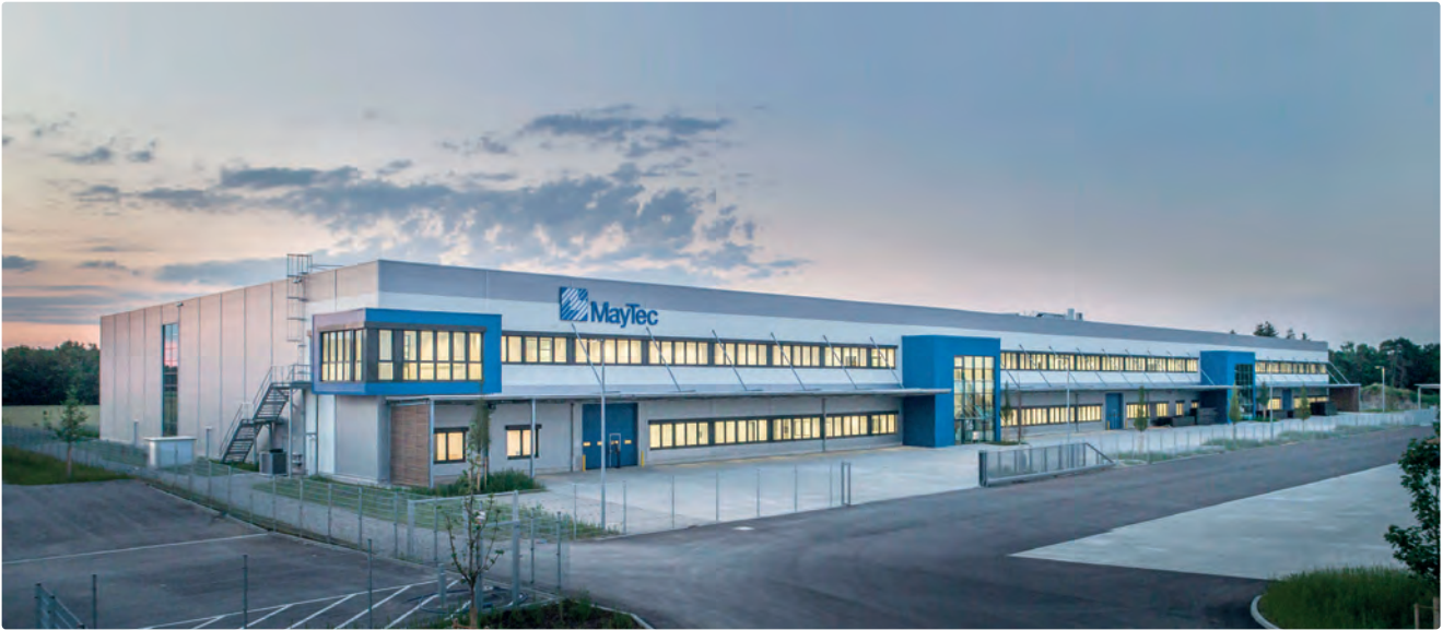
MayTec GmbH plant in Olching
